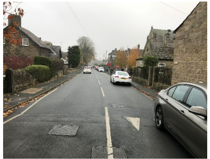
The road at Menston Primary School.
